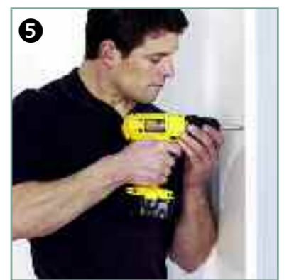
The front edges of the side panels can then be secured to the side wall batons and the fixing screws will be concealed by the door frame.
