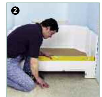
Locate, level and fix the base.
