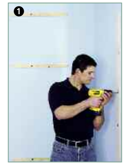
Position and fit the fixing batons to the wall.
