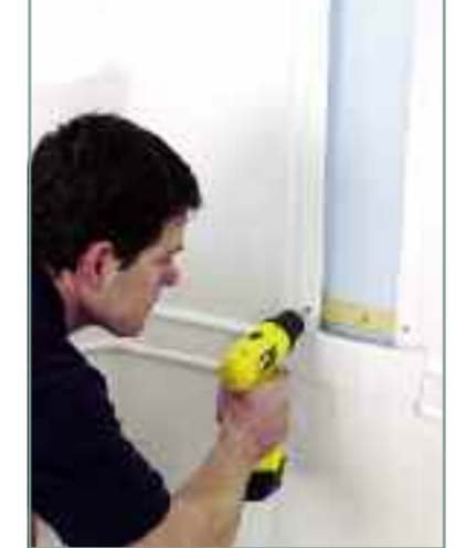
Slot the side panels to the base and fix to the back wall batons, using the spacer provided to ensure that the correct gap is left for the back panel.
