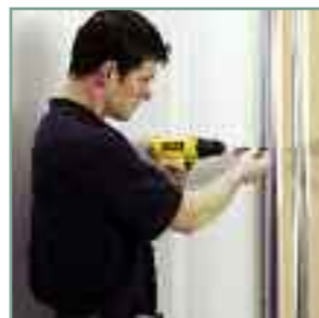
The door is finally secured by drilling through the wall channels into the door frame and fixing with screws.
